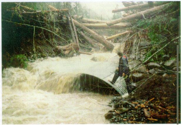
A three-mile long debris torrent swept through Third Creek, a tributary to Fish Creek, and washed out the main road paralleling Fish Creek during the winter of 1995-96.
