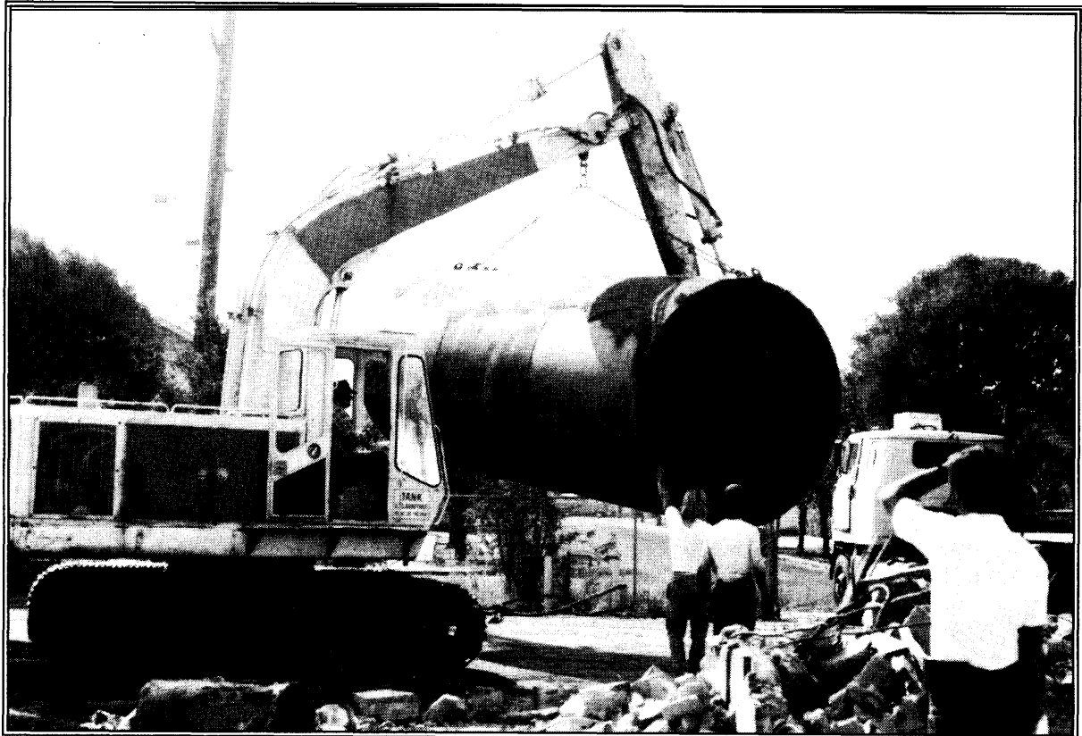
Underground tank removal, 1988 (C. Vath)
